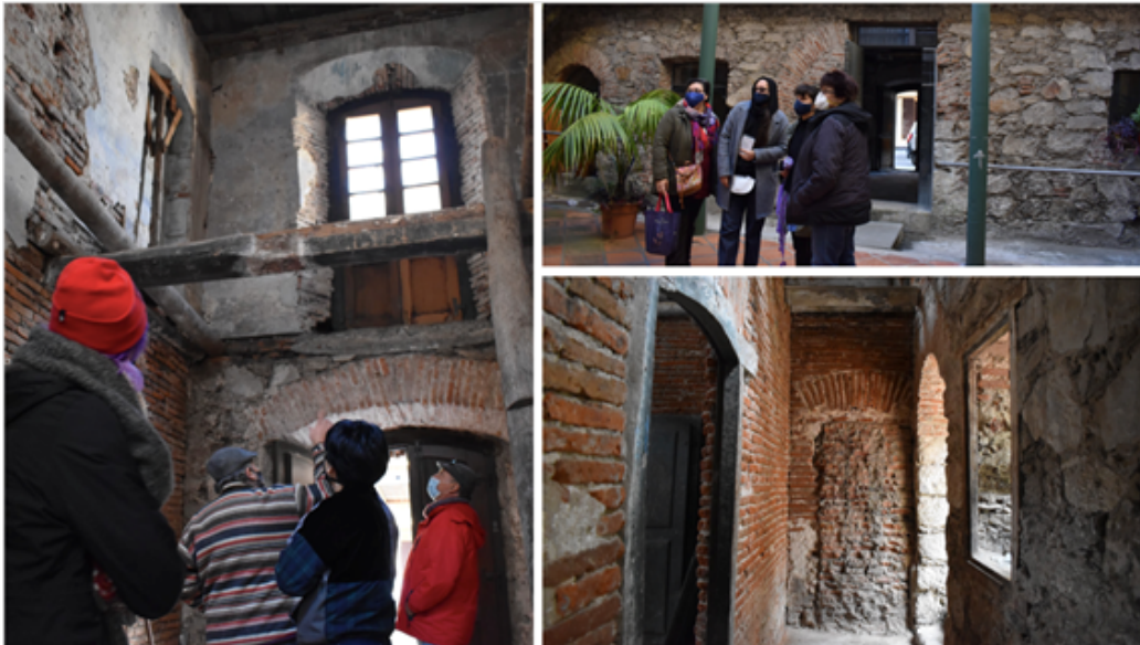
Figure 8: Entry of the groups and architectural evaluation of the state of conservation of Casa de Piedra. 2020. Source: Reactor.
